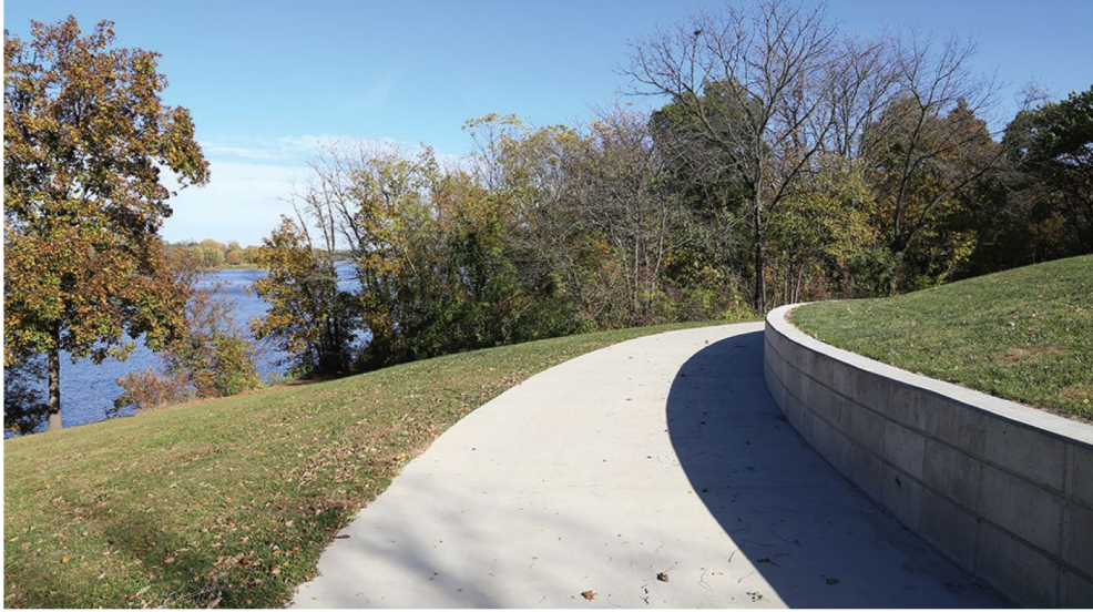
Figure 7-3: Combined retaining wall and trail
