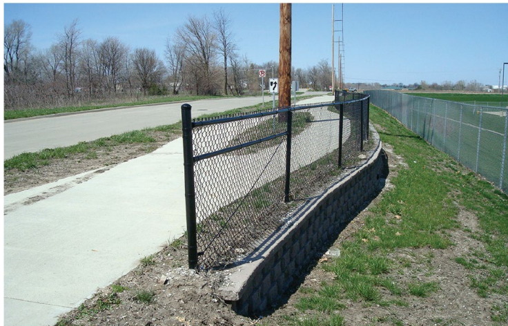
Figure 7-2: Barrier along the trail installed for safety
